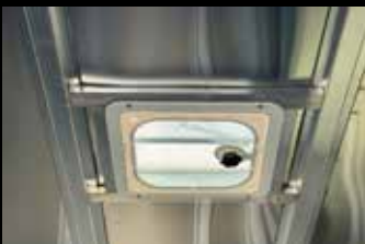
Roof vent in dressing room
